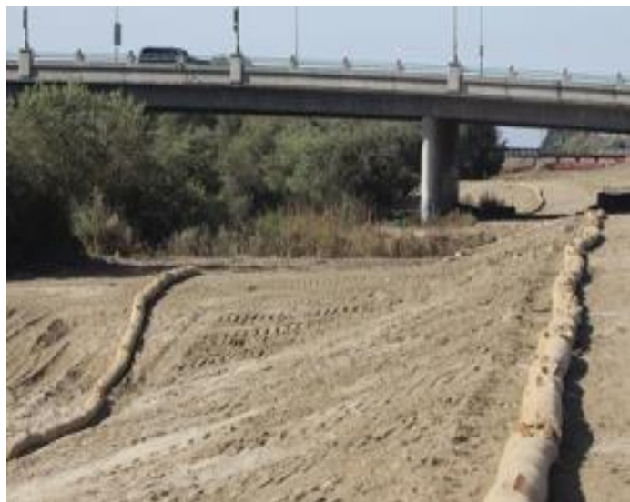
Figure 19: Phase I photo of bench excavation on the Pajaro River.
