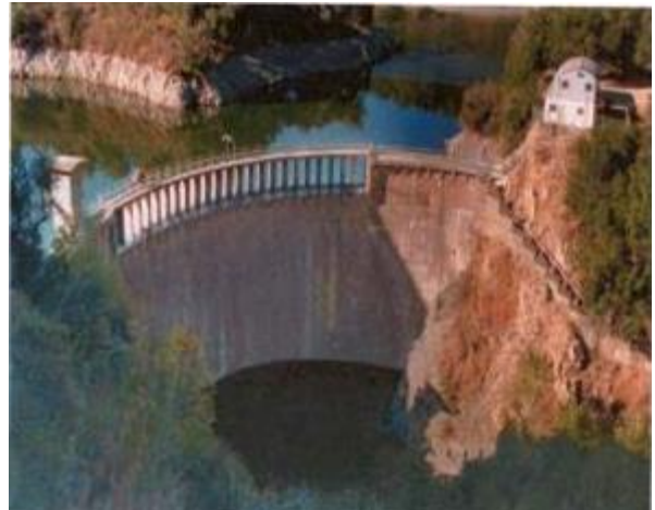
Figure 15: San Clemente Dam
